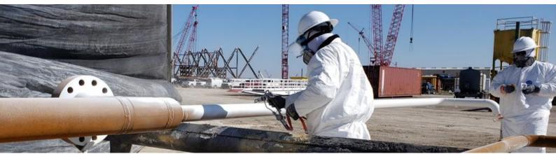
6. Never ever cross contaminate anything between part A and B, that goes for stirrers, brushes, rags, buckets, cleaning water etc. Never the two shall meet!
